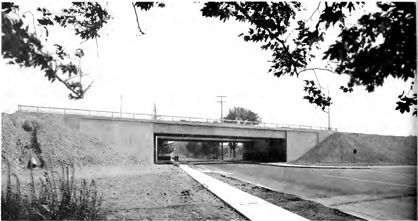
Looking north along Park Avenue showing freeway bridge structure
